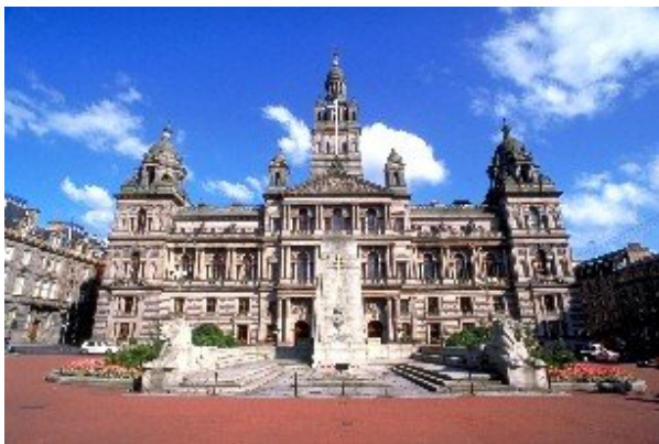
Glasgow City Chambers
